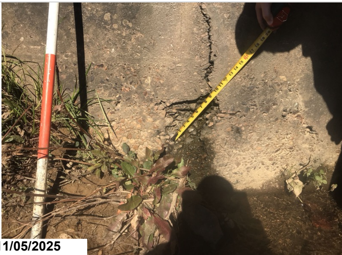
Abutment 1, Right, Under girder 13: 9"X3" deep area of concrete deterioration. 1LF CS3 Spall
