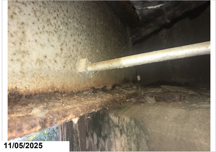
Girder 4, Abutment 2: active corrosion with flaking rust & up to approximately 1/8" section loss. 3LF CS3
