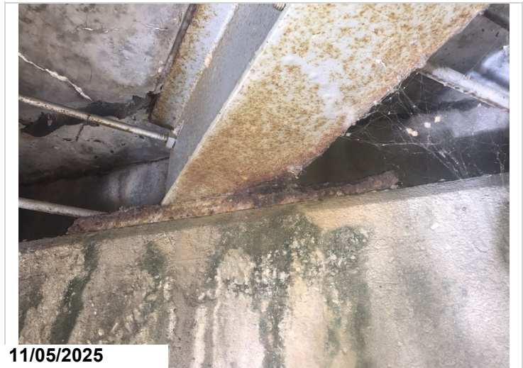
Girder 10, Abutment 1: Active corrosion with flaking rust.
