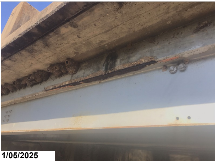
Deck undersurface, Right edge, Adjacent to girder 14: 5' long spall. 5SF CS3
