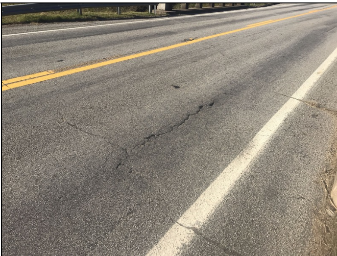
East bridge end: Minor settlement/ rutting.
