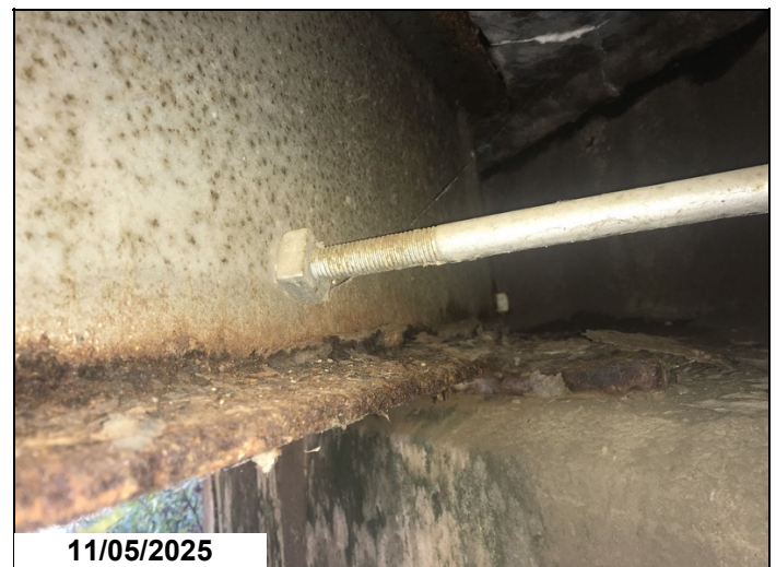
Girder 4, Abutment 2: Active corrosion with flaking rust & up to approximately 1/8" section loss. 3LF CS3
