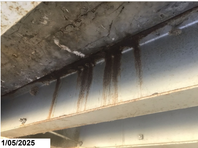
Girder 5, Top flange, Abutment 2: Active corrosion with flaking rust. 4LF CS3
