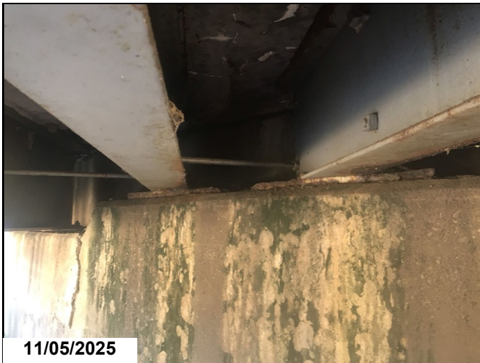
Abutment 2, Bearings: Active corrosion with flaking rust.
