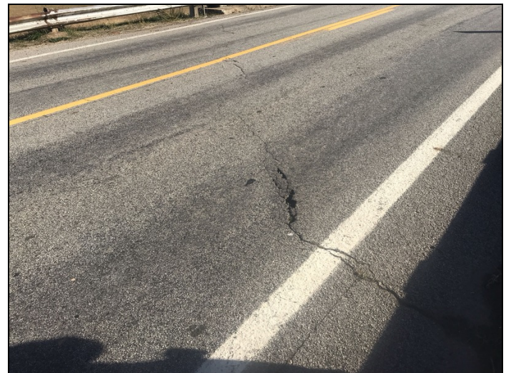
West bridge end: Minor settlement/ rutting.
