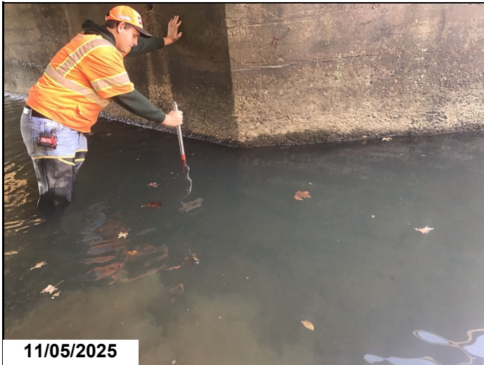
Abutment 1, Left: Top of footing exposed.
