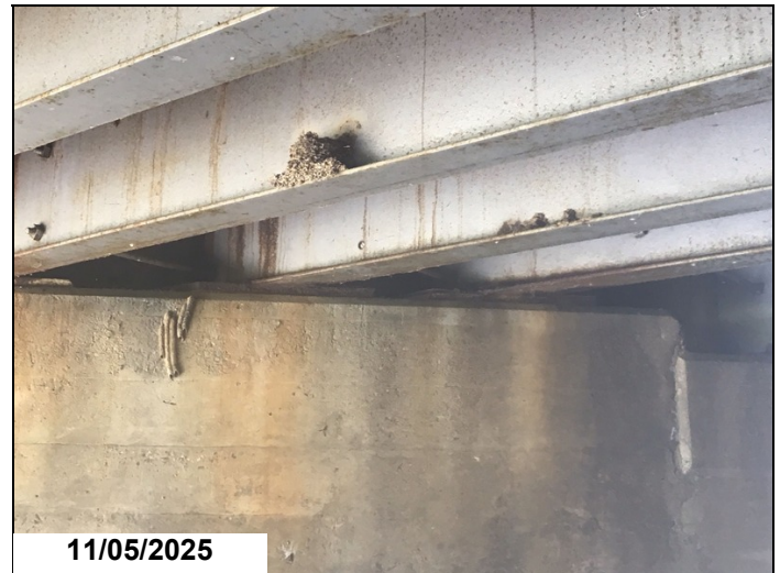
Abutment 1, Bearings: Active corrosion with flaking rust.
