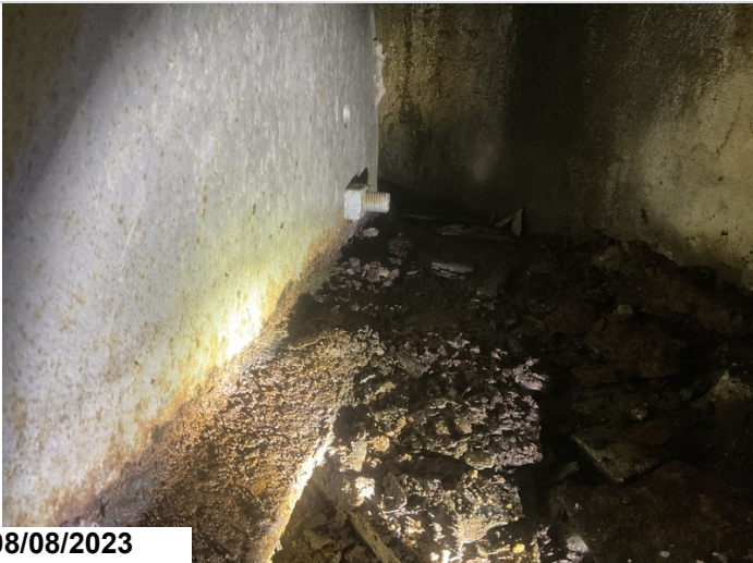
Girders and bearings have a failing paint system with corrosion / section loss.
