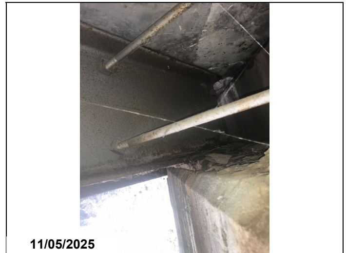
Girder 10, Abutment 1: Active corrosion with flaking rust.
