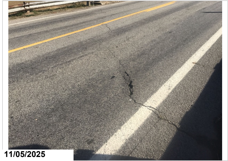
West bridge end: Minor settlement/ rutting.
