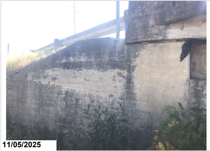
Abutment 2, Left wingwall, Top: Concrete deterioration/ spalling.
