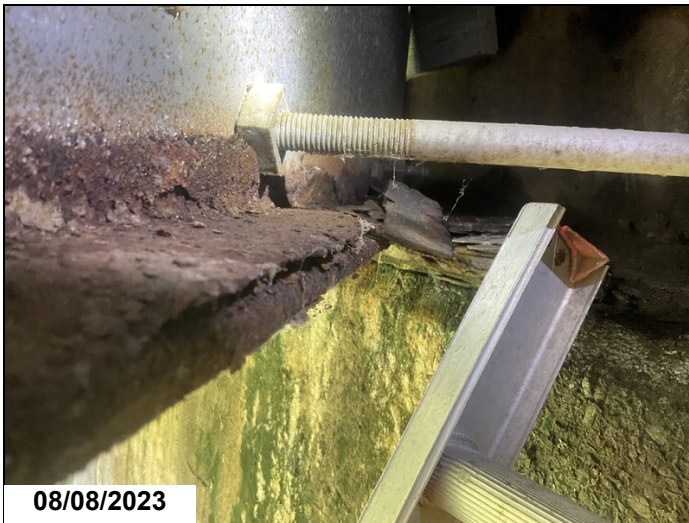
Beam # 11 at abutment # 2-Corrosion with section loss.
