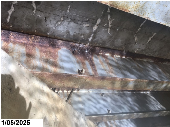
Girder 8, Top flange, Abutment 1: Active corrosion with flaking rust. 10LF CS3
