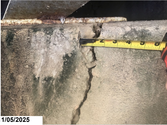
Abutment 1, Under girder 6: Full height vertical crack measures 3/16" at top.
