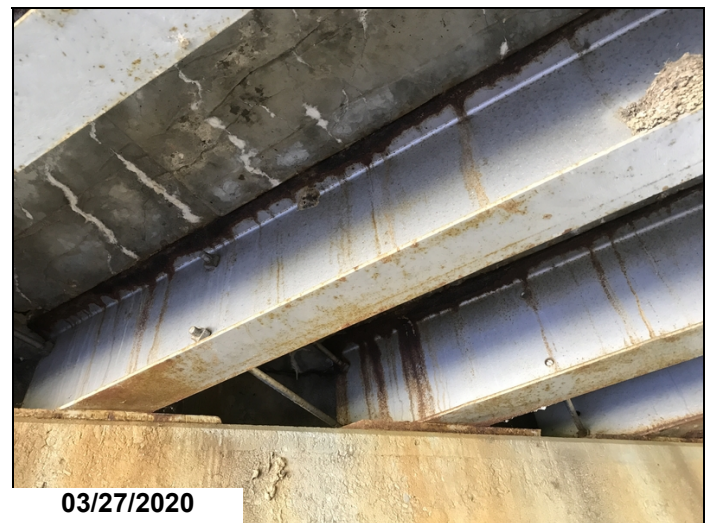
Typical active corrosion along the top flanges in areas.
