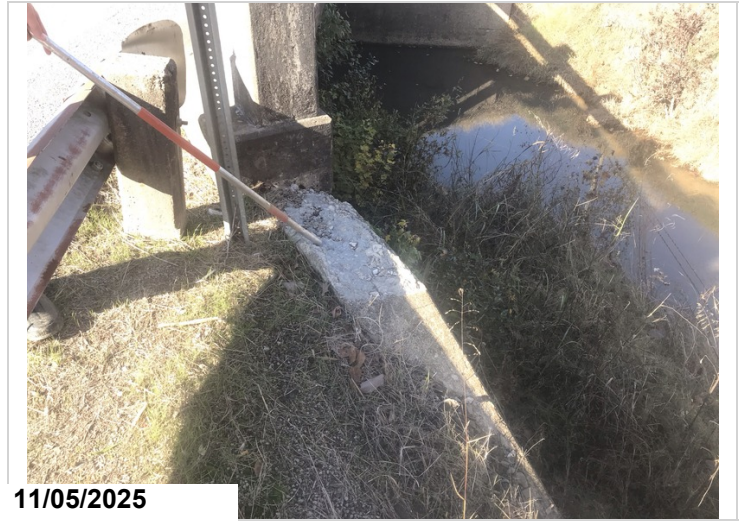
Abutment 2, Left wingwall, Top: Concrete deterioration/ spalling. 3LF CS3
