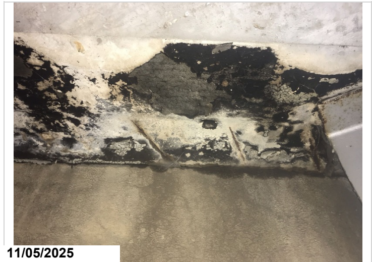
Deck undersurface, Bay 1, Abutment 2: Three shallow 6" spalls with exposed reinforcing steel with initial section loss. 3SF CS3
