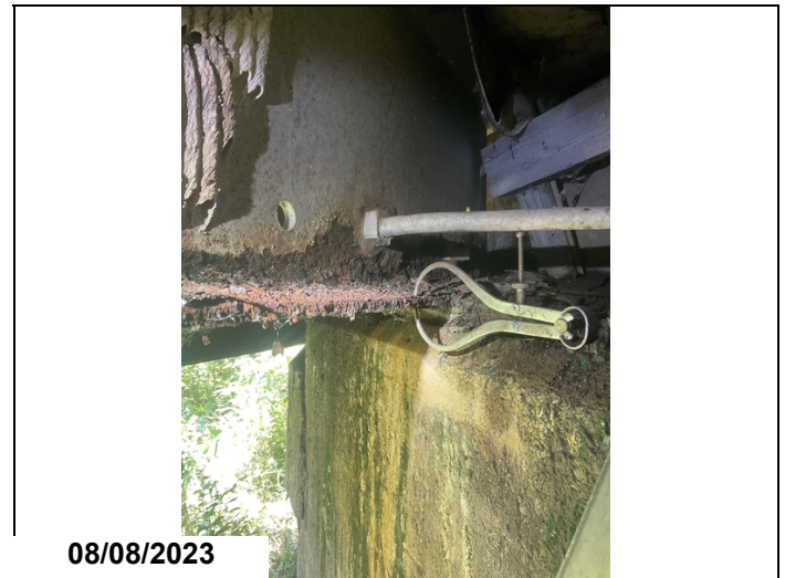
Beam # 12 at abutment # 1 has a 3' long area of corrosion with up to 1/8" section loss with 5/16" remaining section.
