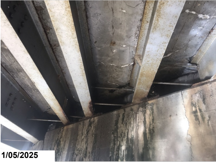
Girders 10, 11, & 12, Abutment 1: Active corrosion with flaking rust.
