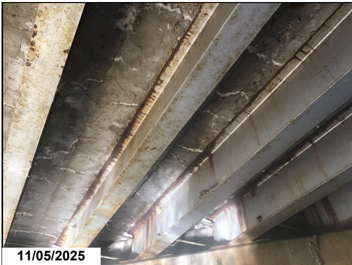
Superstructure, Active corrosion with flaking rust.
