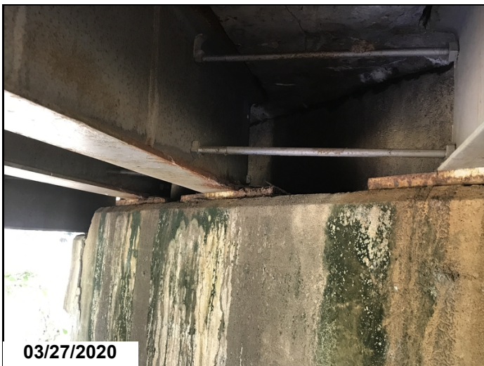
Bearings have active corrosion with pack rust.
